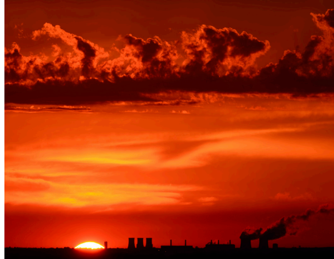
Coal-fired power plant at sunset
